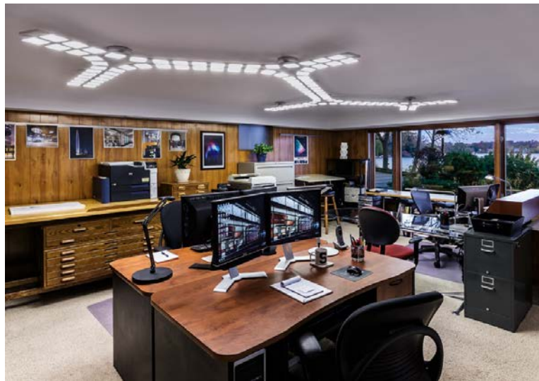
Figure 12. The offices of Aurora Lighting Design with a lighting system using OLED panels. (Photo courtesy of Acuity Brands Lighting)
